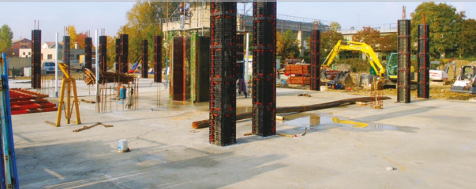
The light, reusable and modular system for the construction of square and rectangular columns
