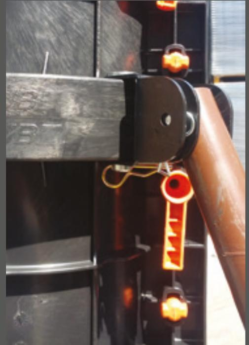
The shoring is performed using a steel bracket to connect push-pull props to the formwork. The brackets are available in various sizes to suit any commercially available props.
